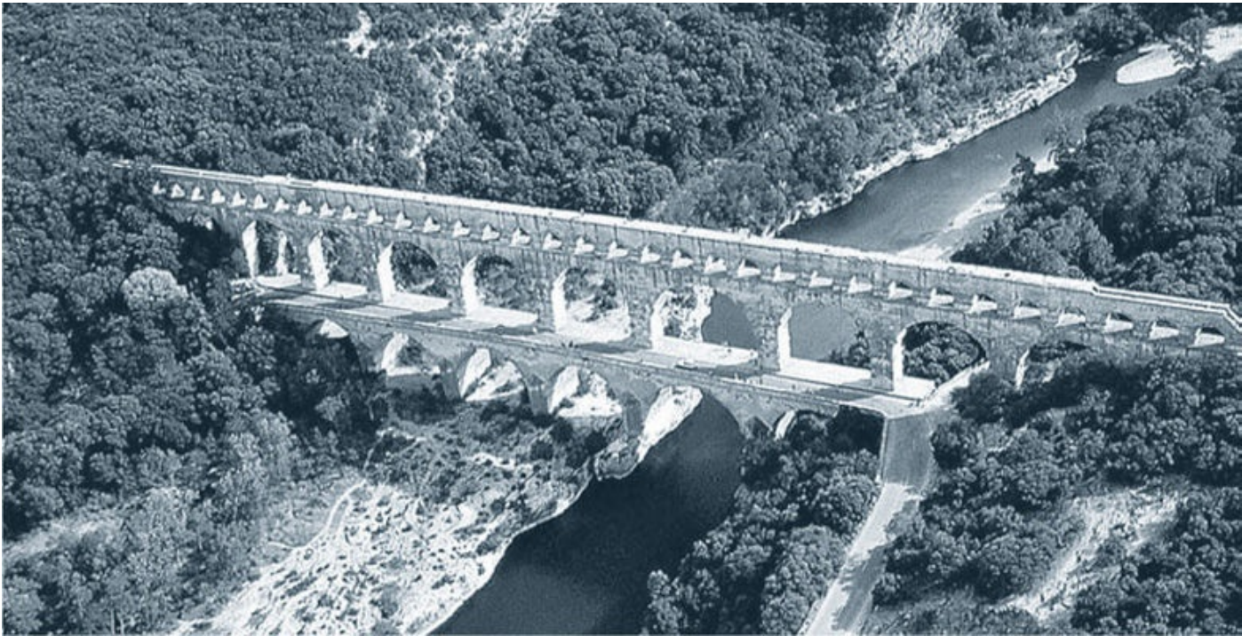
A masterpiece of ancient Roman architecture, the Pont du Gard was built halfway through the 1st century A.D. It is the principal construction in 27-mile-long (50-kilometer), three-level-high limestone aqueducts that supplied the Languedoc-Roussillon city of Nîmes with water.
