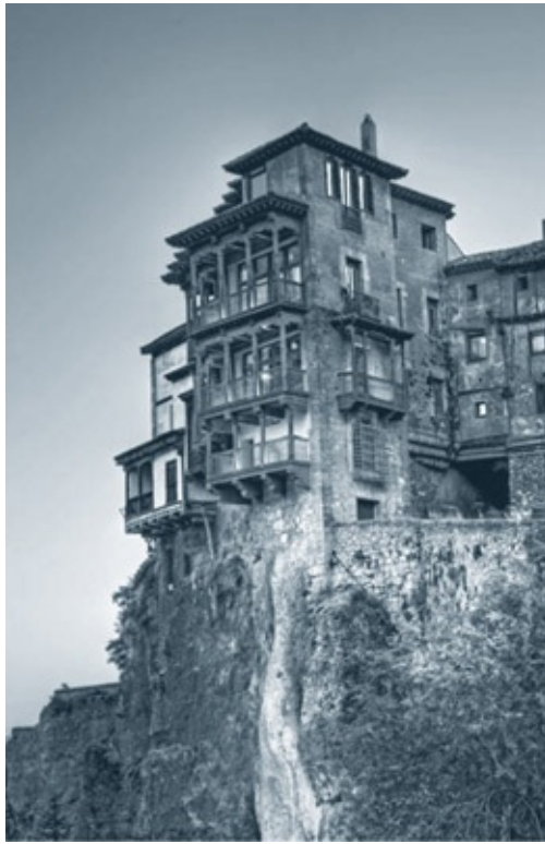
In Castilla-La Mancha, houses cling to the cliffs of the mesata, the vast, rocky plateau of central Spain.
